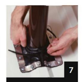
Slide the cable tie through the hole, ensuring that it is resting on the flashing.
