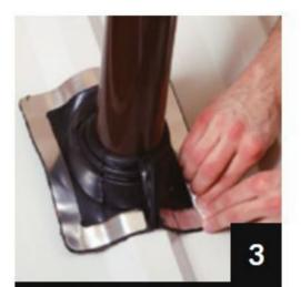
Press Master Flash® Retrofit down, bending it to conform to roof profile or irregularities. A blunt tool will help to form flashing to tight roof angles.
