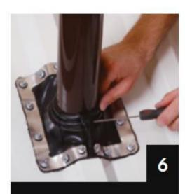
Make a hole in the flange to insert a cable tie or steel band depending on product material.
