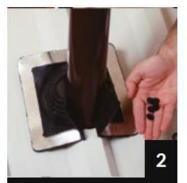
Wrap Master Flash® Retrofit around the pipe and install all snap rivets to seal the flange.
