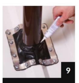
Additional sealant can be applied between the flashing and the pipe.
